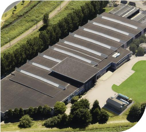
This is Indaver's cutting edge vegetable, garden and fruit (VGF) digester. It is the only machine in South Holland that can both digest and compost vegetable, garden and fruit waste, green waste and biowaste from the food industry and processes organic waste into green gas for around 3,000 households. Indaver recovers three valuable products from the process: compost, green gas and liquid CO<sub>2</sub>.
