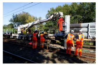
Figure 51: Piling train arrangement
