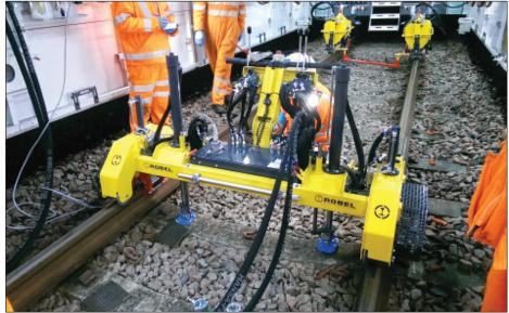
which can be installed without the need to lift or slew the conductor rail. The obvious advantages are that we remove the risk of leaving the conductor rail up on the insulator pots and remove the danger of crushing injuries to staff.'
