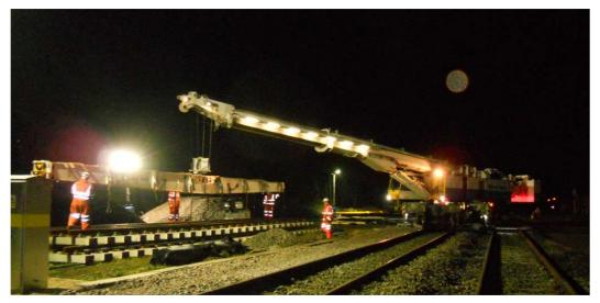
Figure 48: Kirow 1200 lifting S&C Panels
