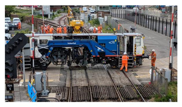
The Beaver tamper is rotated on a pivot at the middle of the machine as seen in the photograph. The workers can then push it round facing the right direction.
