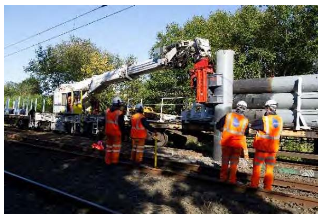
Figure 51: Piling train arrangement
