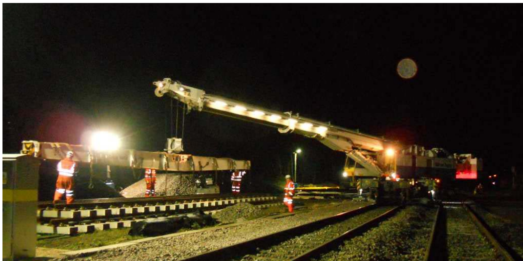
Figure 48: Kirow 1200 lifting S&C Panels
