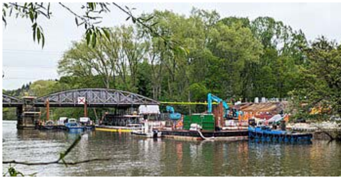
Nuneham Viaduct repair from downstream with south span supported and south abutment removed
