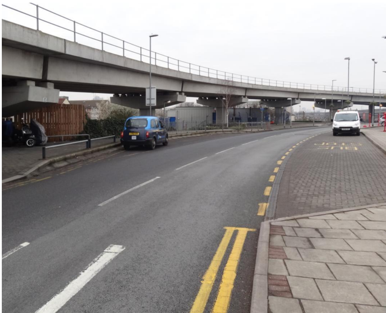
Figure 1 - Potential for restricted visibility at new zebra crossing
