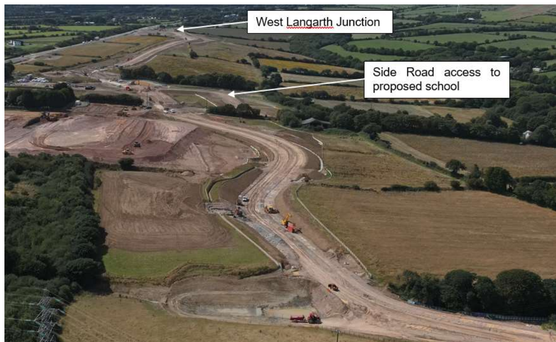
Figure 11 - showing the eastern extent of the NAR earthworks and the formation of the side road towards Little Treworder Farm (photo taken in October 2023).
