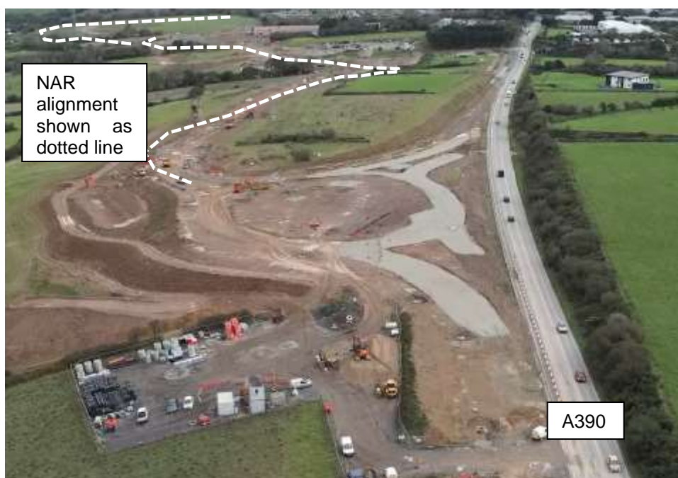
Figure 9 - West Langarth Junction, looking east, showing earthworks completed and drainage works starting (photo taken on 25 October 2023)
