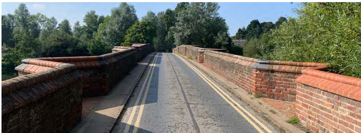
Figure 6.8: Photograph showing lack of NMU facilities at Clifton Hampden Bridge
