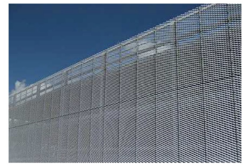
5 Expanded aluminium mesh Image of expanded aluminium mesh with trapezoidal eye slits cladding system showing top section of the facade without any backing panel
