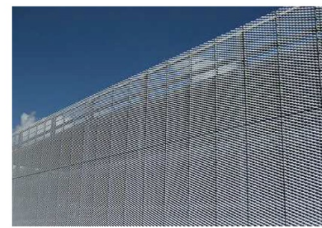
5 Expanded aluminium mesh Image of expanded aluminium mesh with trapezoidal eye slits cladding system showing top section of the facade without any backing panel
