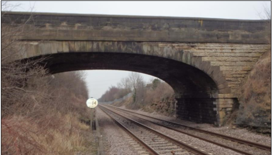
Figure 25: Existing Ridge Road basket arch design.
