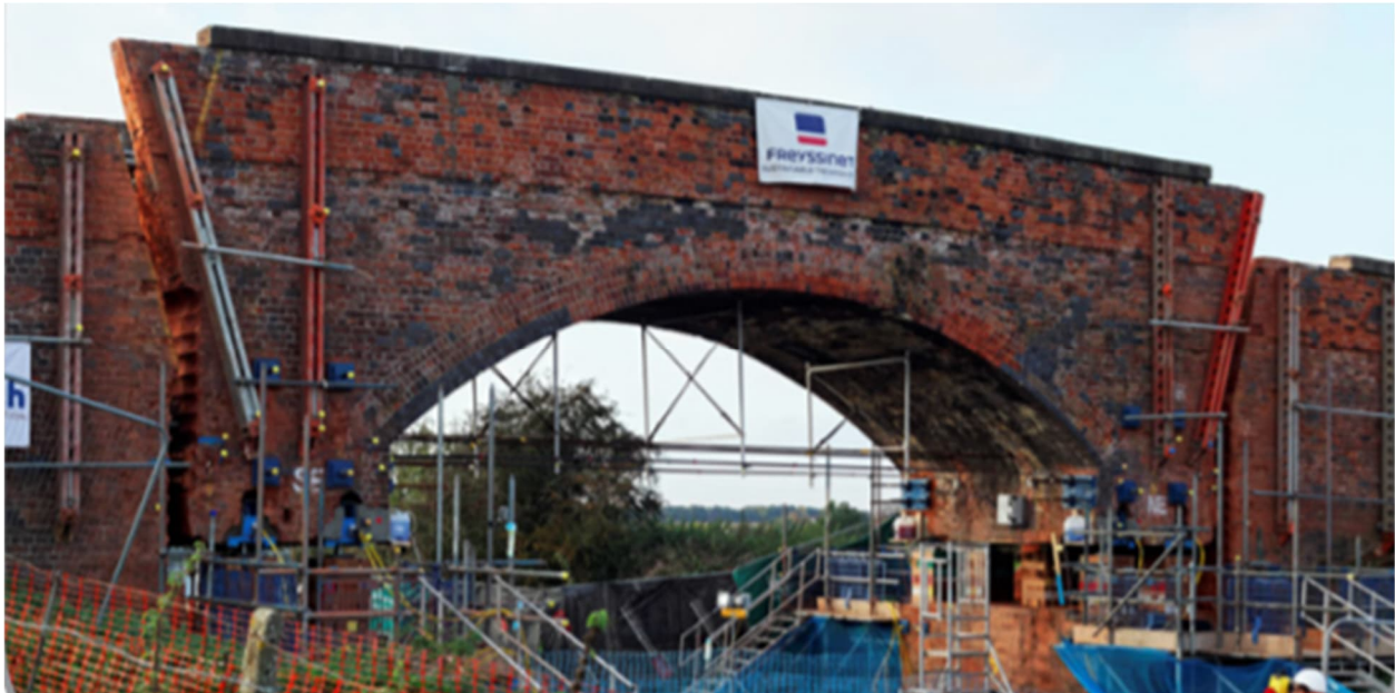
Figure 7 – Trial brick arch jacking site Moco Farm
