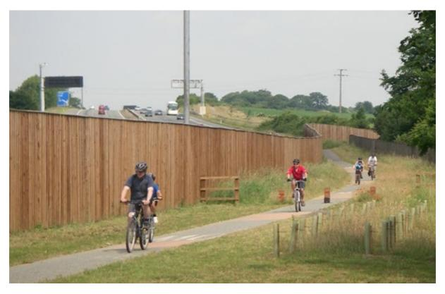
Figure 31: 3.0m Two-way Cycle Track with Barrier Layout
