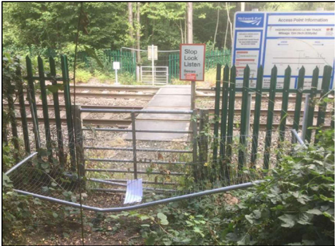
Highroyds Wood Level Crossing showing vandalised temporary fencing
