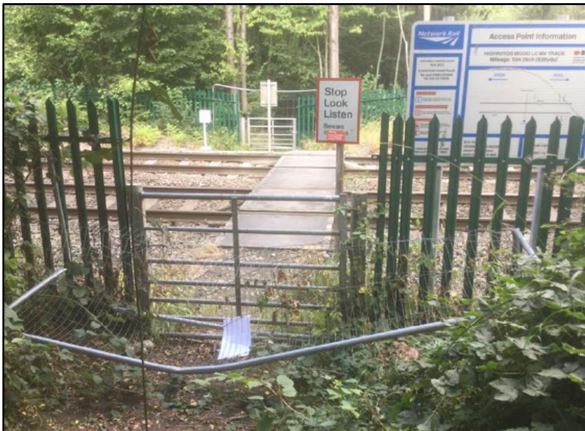
Figure 8: An image of the temporarily closed Highroyds Wood Level Crossing showing how the temporary fencing had itself been vandalised
